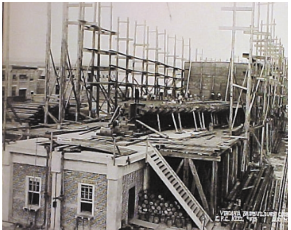
This photograph shows how the shipway and scaffolding supported the keel and hull and provided work platforms for rivet gangs and other workers. As each level of hull was built, a new layer of wooden scaffolding was added.
